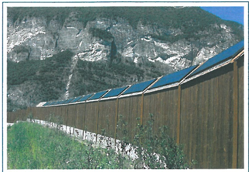
Fig. 7 - North-South orientation of the sound absorbing structure in relation to the daily path of the sun
