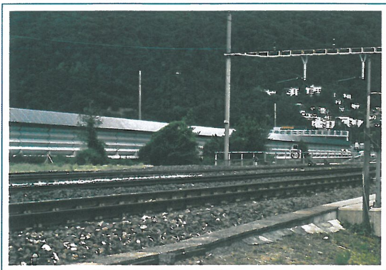
Fig 5 - Acoustic barrier integrated with photovoltaic panels alongside the railway line that follows the A1 motorway close to Lugano, in Switzerland
